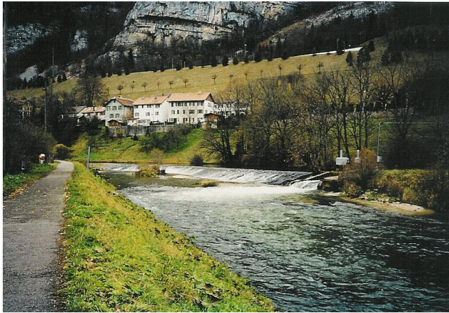
Photo 1. Weir on the Orbe river with the intake on the left bank, at Vallorbe, Switzerland
